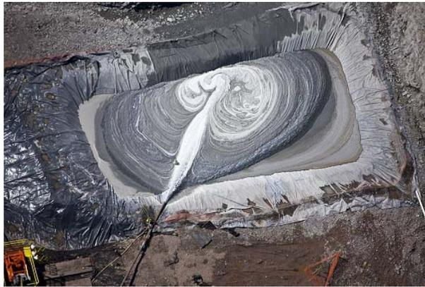
Waste pit for toxic drilling fluids...note the overspray as well.
